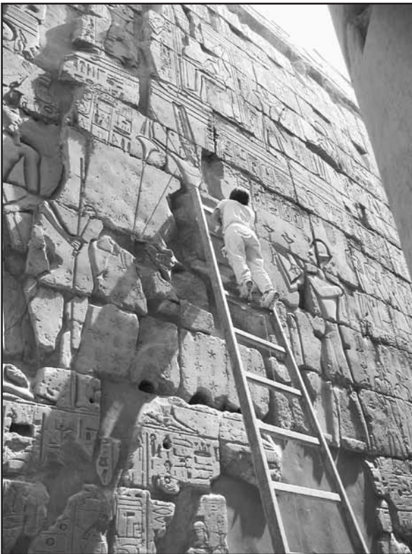
Figure 12. Hiroko installing a plumb bob monitor halfway up the south face of the east pylon, Luxor Temple. Luxor, Egypt. Photograph by Ray Johnson
