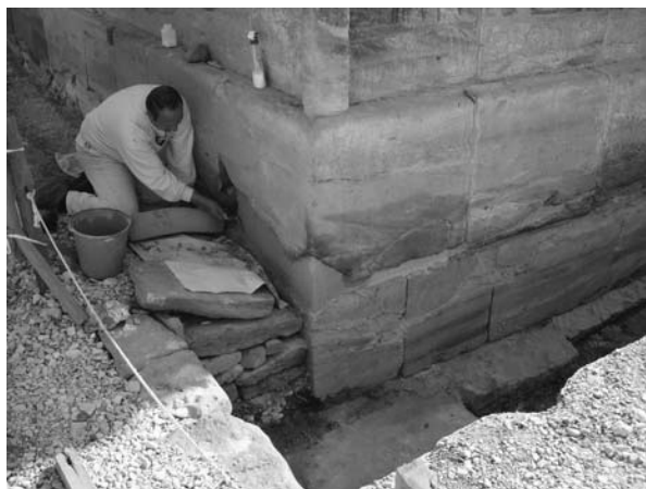
Consolidation and infilling the outer southwestern wall of the small Amun temple sanctuary. Photo by Ray Johnson
