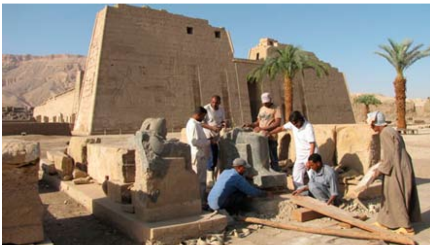
Figure 5. Lotfi and team moving material to the new blockyard. Photo by Nahed Samir
