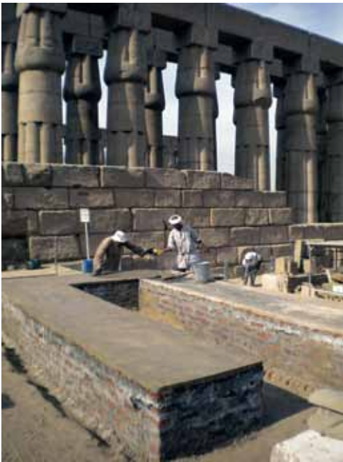
Display mastaba finishing
