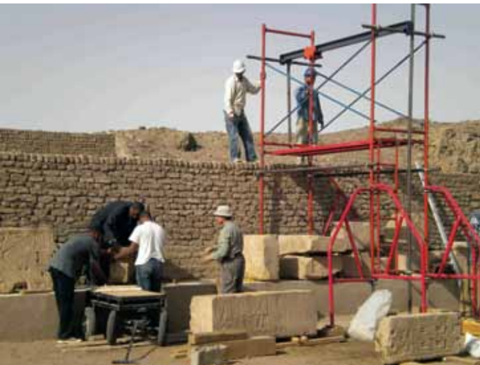
Medinet Habu blockyard block moving by Frank and crew
