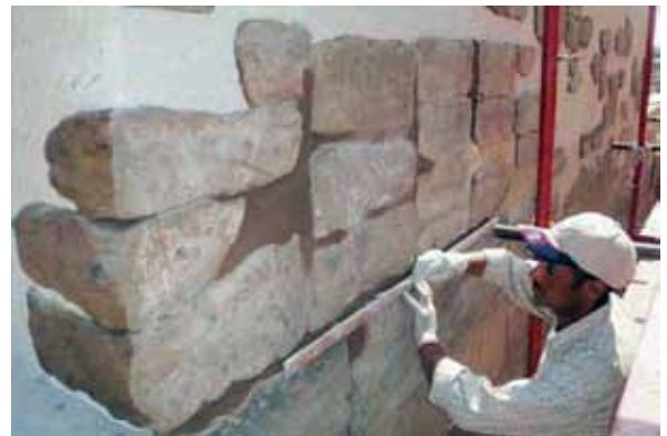
Amenhotep III wall being plastered and infilled by Salah
