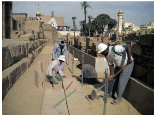
Luxor Temple blockyard open-air museum path construction
