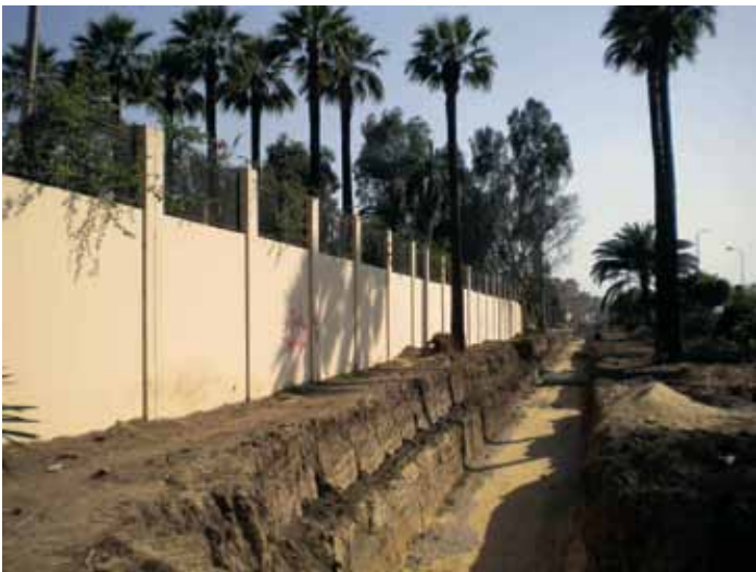
Service tunnel trench outside Chicago House, March 24, 2010
