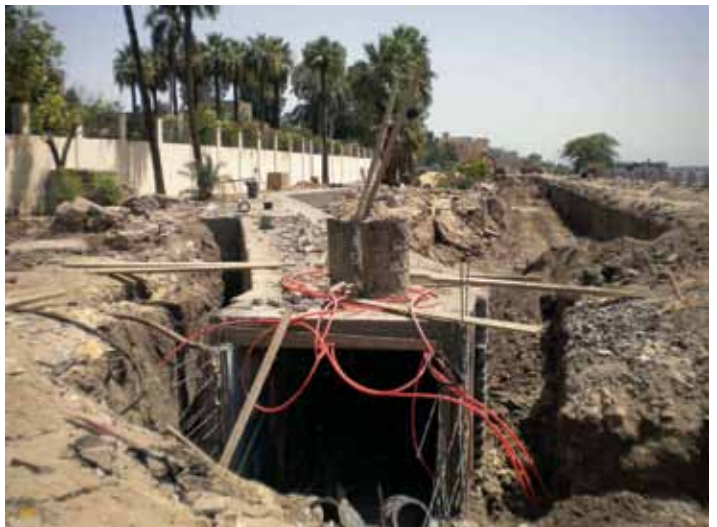
Corniche service tunnel and riverbank construction, June 2010
