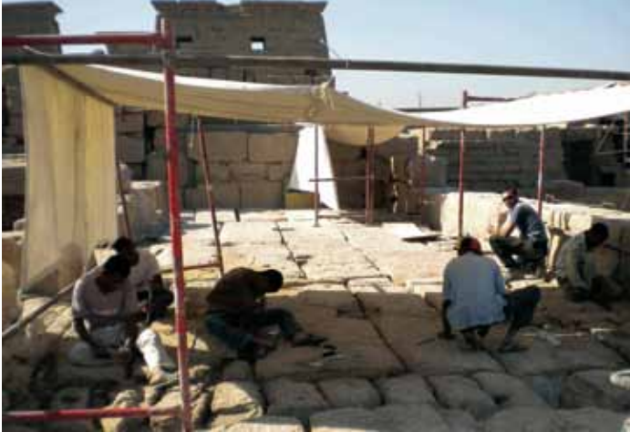
Khonsu Temple roof work
