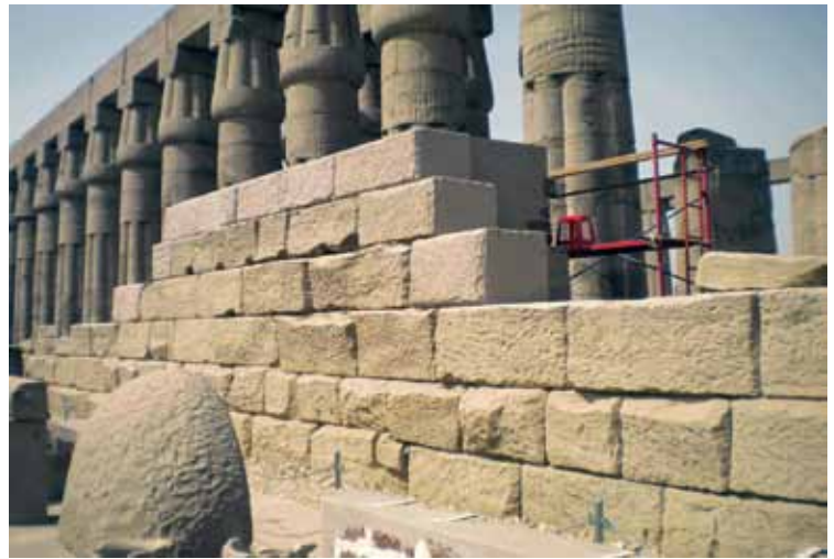
Amenhotep III outer wall finished
