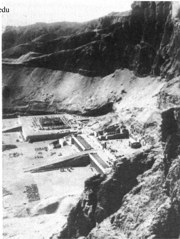
Fig. 19b.—The Deir el-Bahri Bay, with Hat-shepsut's Temple in the Foreground and Mentu-hotep's in the Background
