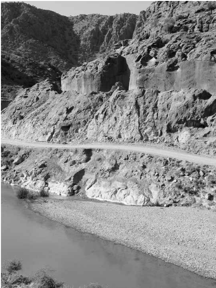
Figure 3.2. The most impressive section of the rock-cut canal (“road”), on the right bank of the Tang-i Bulaghi. The passage follows the steep slope for over 250 meters, about 15 meters above the Pulvar riverbed
