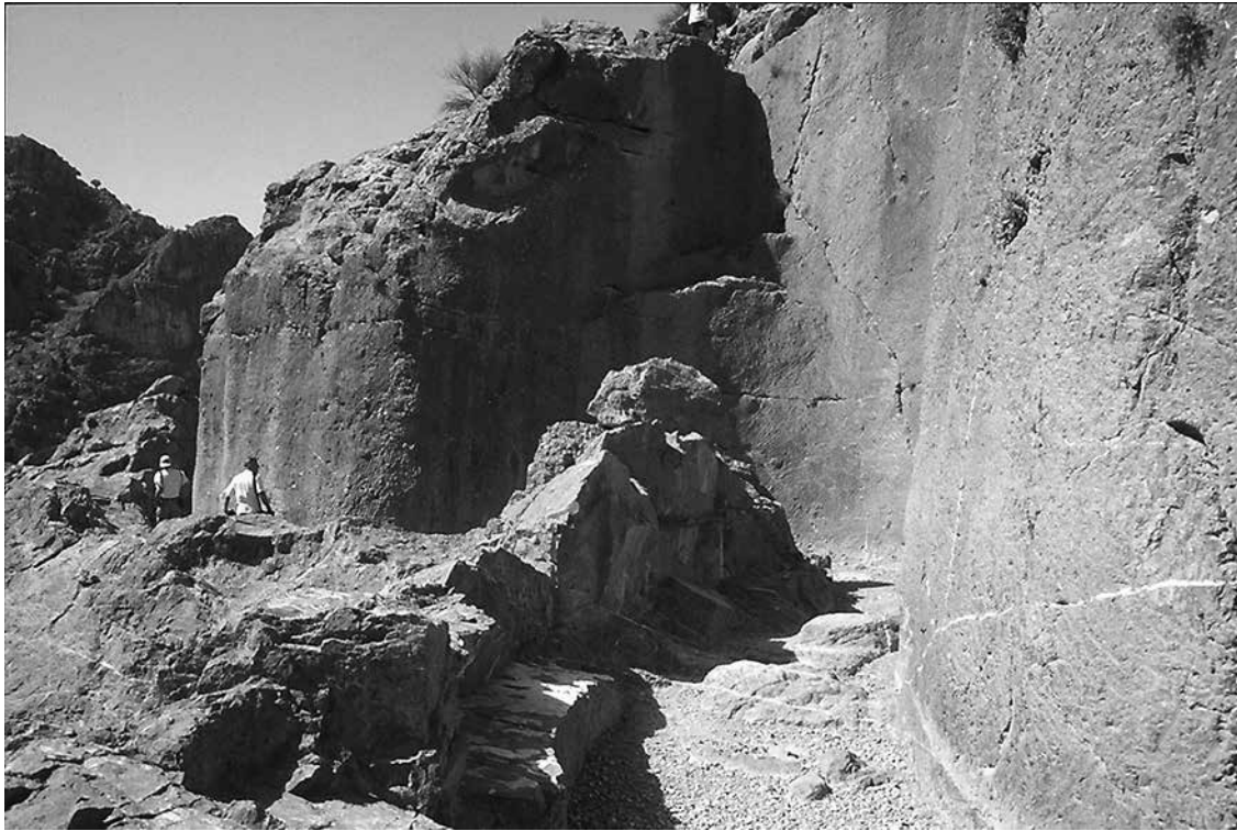
Figure 3.3. Detail of the canal, about 1.5 meters wide. In the curve it has been cut down to a depth of 10 meters
