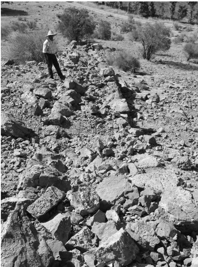
Figure 3.4. A stone-built section of the canal. The 2.5-meter wide “wall” made of two rows of boulders with a filling of pebbles likely represents the substructure of the canal itself
