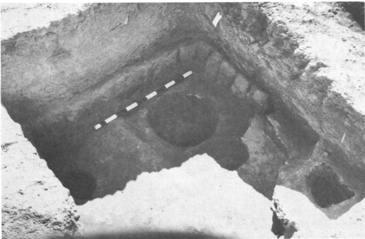
FIG. 8.—ROOM 33, PROBABLY USED FOR WASHING, SHOWING DAMP COURSE AND SUNKEN RECEPTACLE FOR WATER IN THE CORNER PLATFORM ON THE RIGHT
