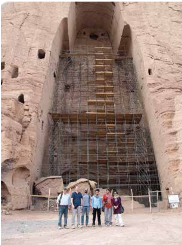
Figure 9. The OI team in front of the empty niche that once held the larger standing Buddha of Bamiyan. UNESCO conservators have erected scaffolding inside the niche as part of their efforts to stabilize it and prevent further collapse
