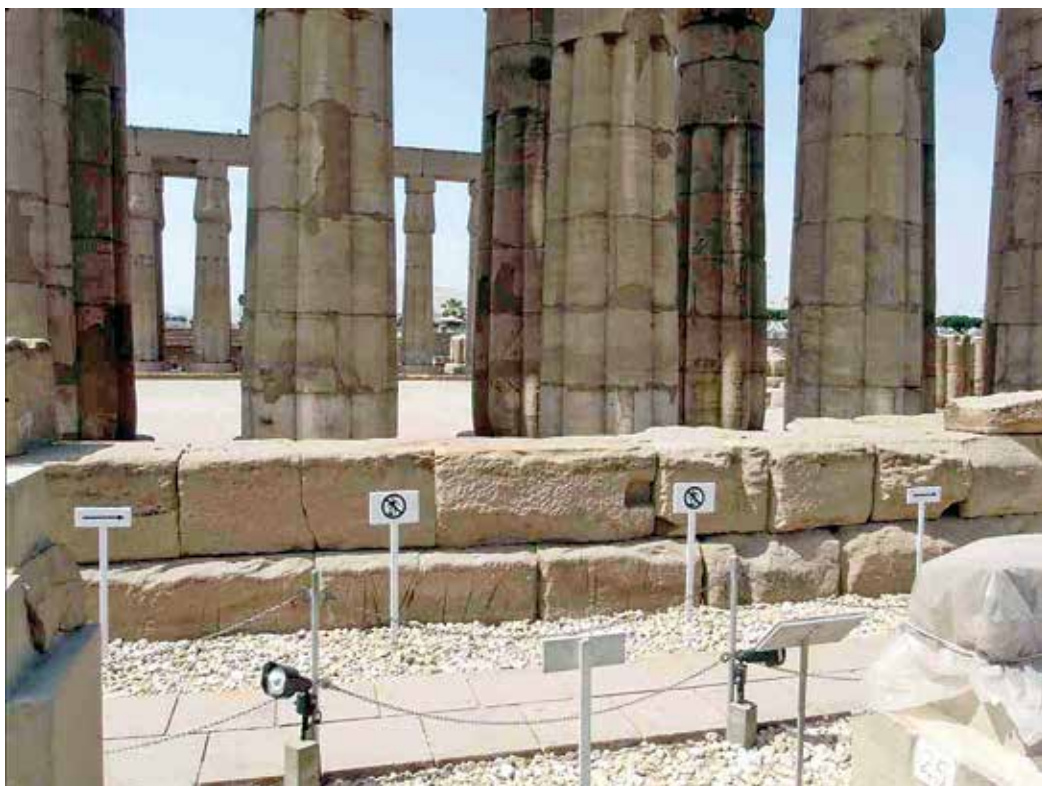
Figure 14. Newly installed “do not climb” signs for the walls of the Amenhotep III court (photo by Ray Johnson)
