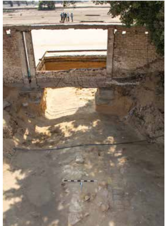
Figure 3. The west RAB wall continuing below the Abu Hol Sports Club; view to the south.
