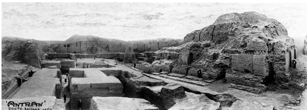
Figure 21.4. Nippur Area EN in 1950. The view is from the north side of the Ekur—the temple complex of Enlil—toward the south, with the temple in the foreground (left, or east) and the ziggurat of Enlil in the background (right, or west). ISACM P. 47787.
