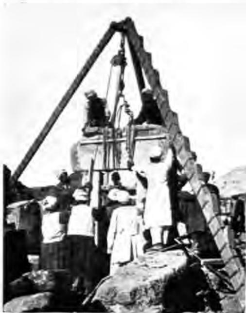
FIG. 82.—RE-ERECTION OF A FALLEN LINTEL IN THE HAREM
