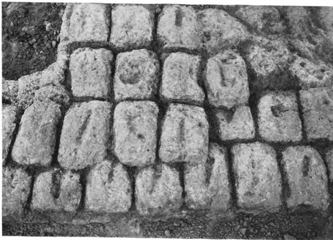
FIG. 14.—Bonded brickwork (of unbaked bricks) in a wall at Khafaje
