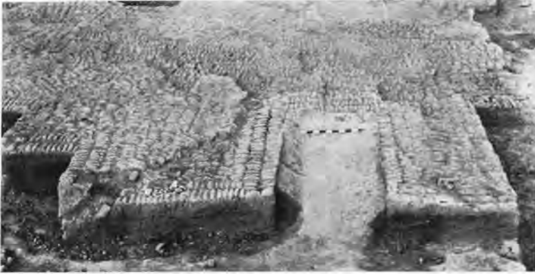
FIG. 16.—Typical brickwork (of unbaked bricks) at Khafaje, marking the outer face of the recessed towers (left) flanking the entrance and of the gateway and gate chamber (under measuring stick).
