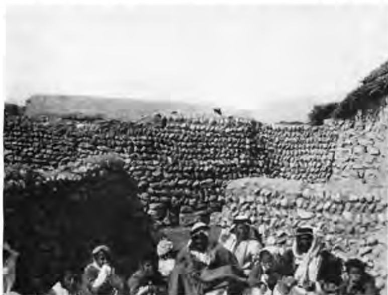
FIG. 24.—Modern stone houses in northern Iraq showing herringbone pattern in the wall structure.
