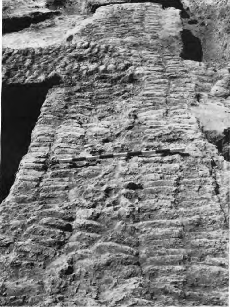
FIG. 25.—A wall of crude bricks at Khafaje. Two rows of regularly laid bricks on each side with irregularly laid bricks between them. Note the difference in structure where this wall and the one in background meet.
