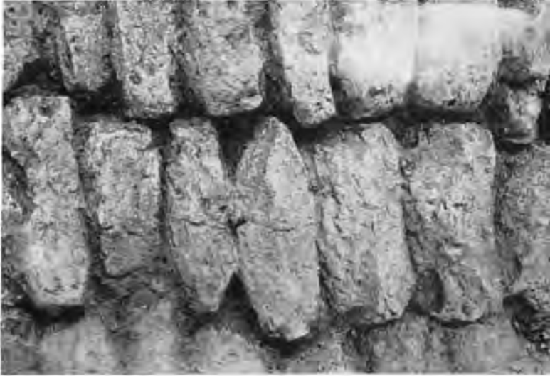
FIG. 3.—Unbaked plano-convex bricks of different sizes used in the same wall at Khafaje.
