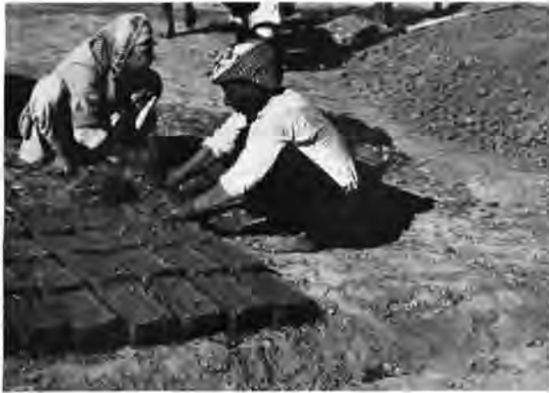
FIG. 2.—Brickmaker removing surplus of clay projecting above frame
