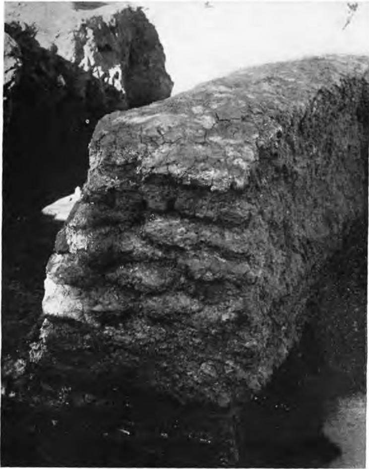
FIG. 15.—Bonded brickwork (of unbaked bricks) at the corner of a wall at Khafaje.
