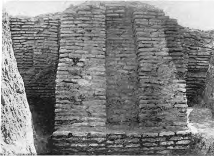
FIG. 13.—Buttressed drain at al-Ubaid showing bonded brickwork
