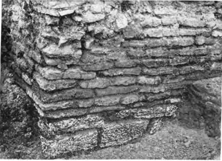
FIG. 12.—The corner of the retaining wall at al-Ubaid, built over a stone foundation and bonded by means of alternate headers and stretchers.
