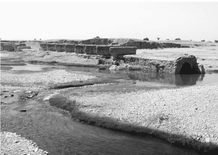
The siphon-bridge at Jundi-Shapur
