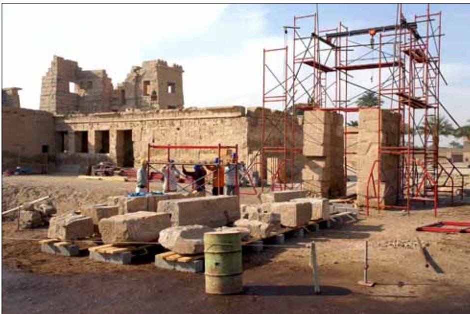
Figure 2. Domitian gate dismantling, March 3, 2011. Photo by Ray Johnson
