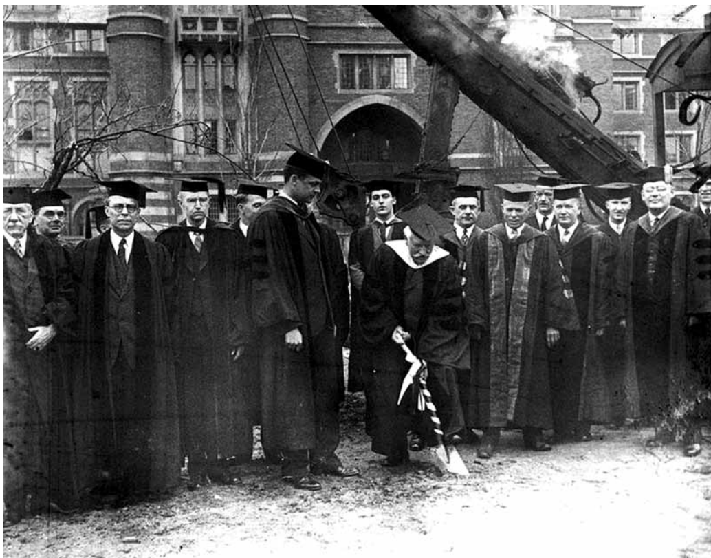
Groundbreaking ceremony for the Oriental Institute, archival photographic files apf2-05471, Special Collections Research Center, University of Chicago Library
