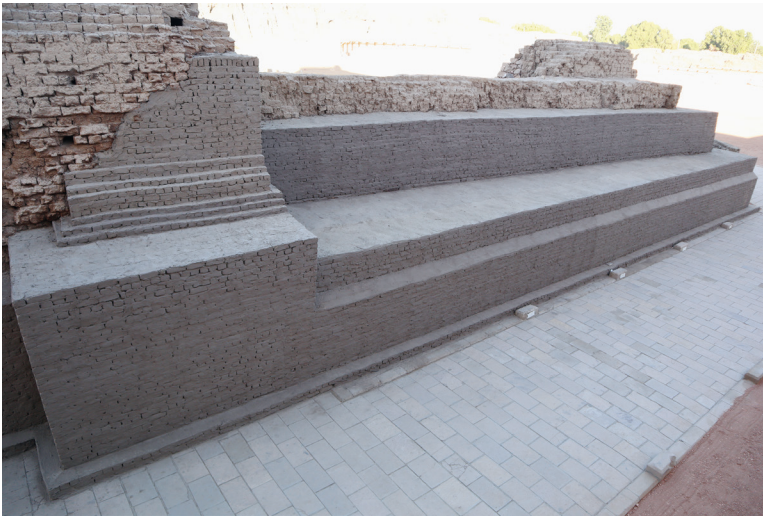
LEFT: Figure 20. New protective mudbrick wall constructed on the eastern side of the Ptolemaic enclosure wall. Photo: G. Marouard, Tell Edfu Project.
