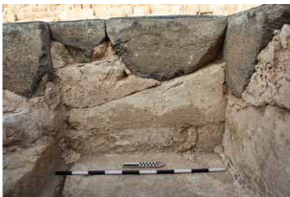
Figure 3. Basalt pavement slabs set over underlayer of limestone cut to conform to the bottoms of the slabs. Photo by Dan Jones.
