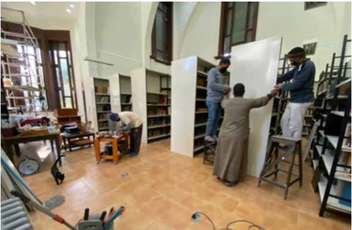
Figure 27. Chicago House Library Second Hall, reassembly of bookshelves. Photograph by Tina Di Cerbo.
