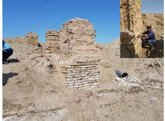
Figure 1. Restoration of the columns of the Parthian monumental building at Nippur.
