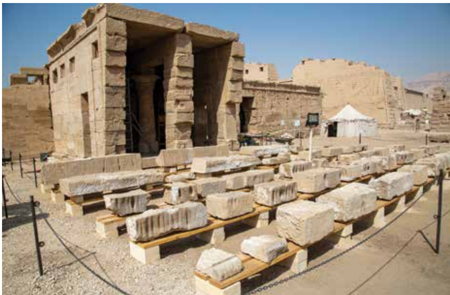
Figure 11. Dismantled Taharqa Gate blocks prepared for conservation, April 2022. Photo by Frank Helmholz.
