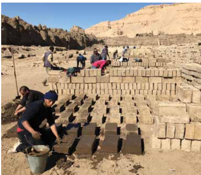
Figure 12. Manufacturing new mudbricks with molds, January 2022. Photo by Ray Johnson.
