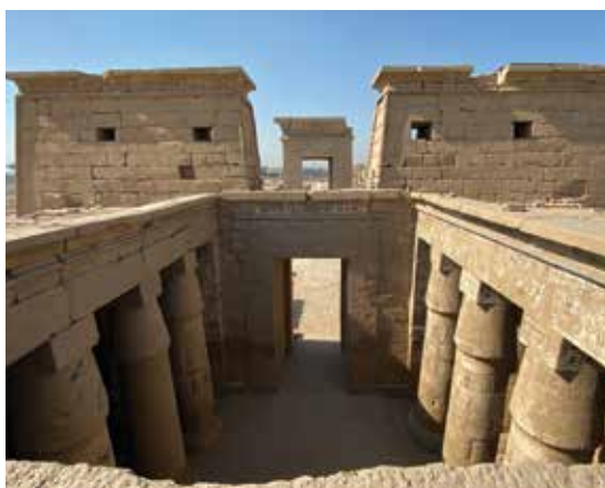
Figure 30. View toward the south from the roof of Khonsu Temple. Photo by Ray Johnson.
