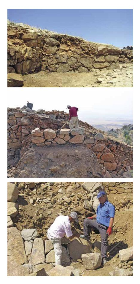
$(\alpha)$  The intensity of the fire caused some facing stones to lose their structural integrity and load-bearing capacity; these stones are fragile and are easily fragmented into small pieces, further dislocating the rubble infill behind them.
