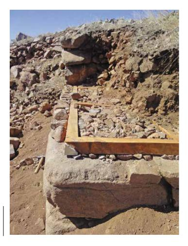
(a) The horizontal timber beams were located ca. 5-10 cm inside the wall faces, as they were in the original masonry, so that they would not be visible from the surface and prone to rapid deterioration.
