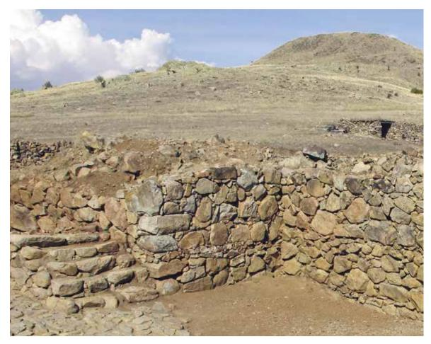
(  $\alpha)$  At the North Tower the wall top was raised to the level of the adjoining walls.
