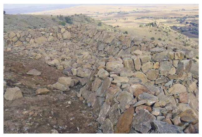
( $\alpha$ ) As a safety measure, the restored tower walls were raised to form a parapet to prevent visitors from walking too near the edge.
