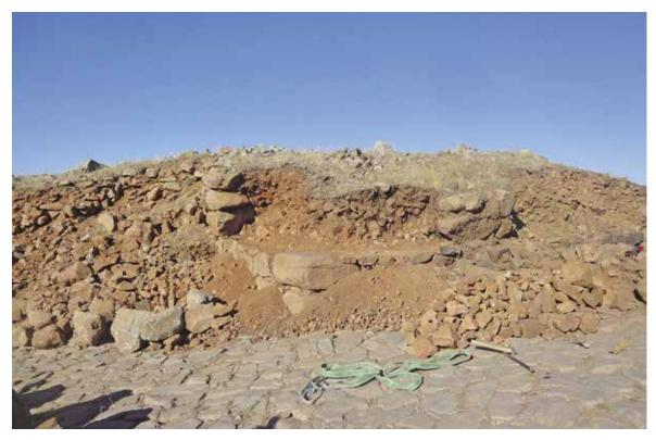
(b) The southern and eastern faces of the West Tower were dismantled down to the level of the horizontal timber beam.
