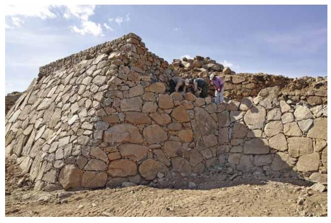
( $\alpha$ ) The southeastern corner of the East Tower was rebuilt with comparatively smaller stones that can be distinguished from original work.
