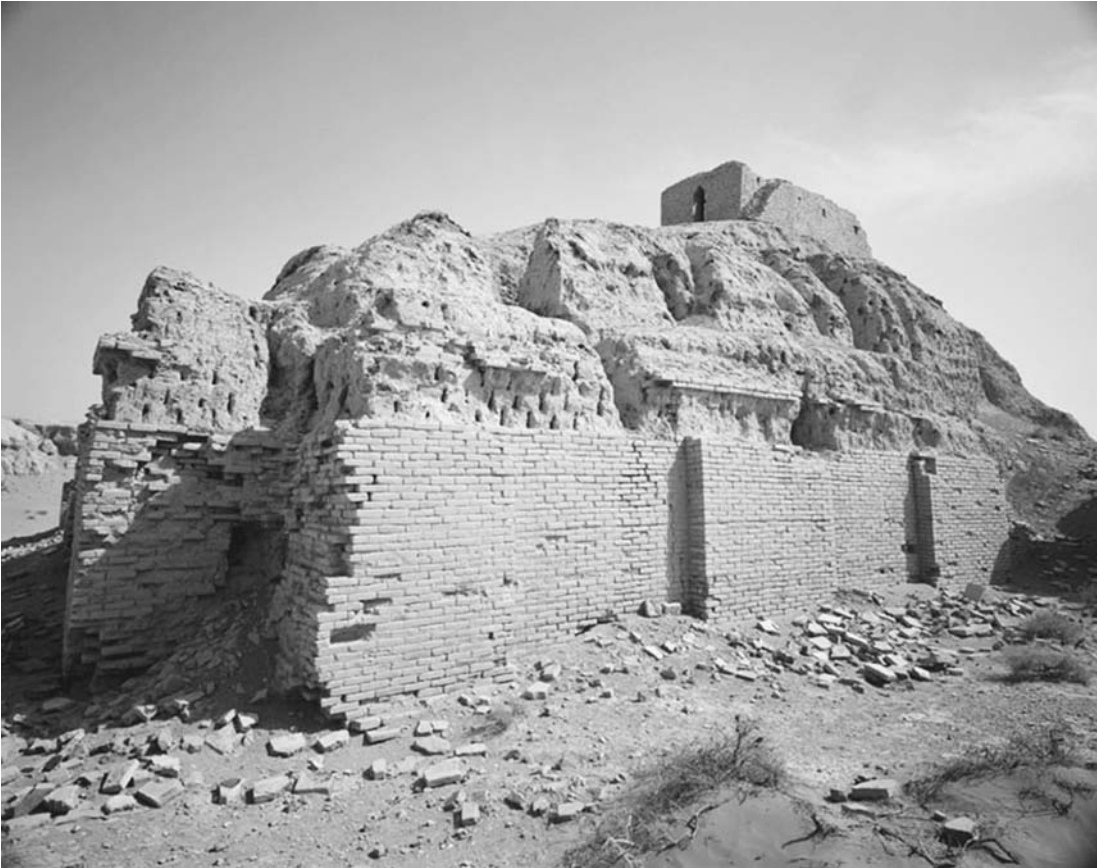
Nippur Ziggurat showing damage to Ashurbanipal baked brick façade. Looters remove bricks to look for those inscribed and discard those without inscriptions
