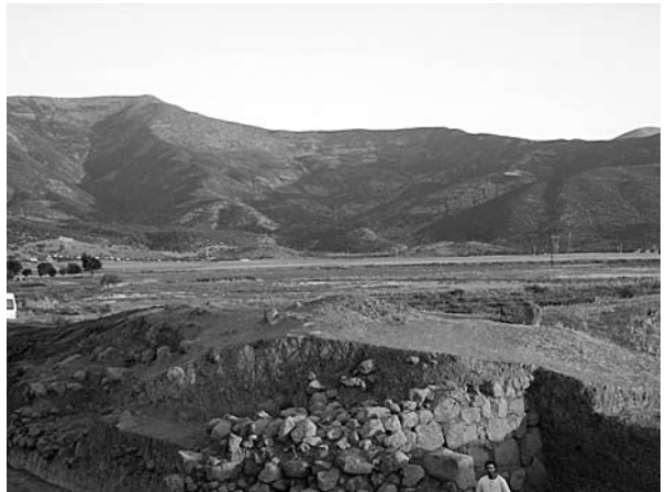
A modern canal has cut through the Iron Age city wall on the southeastern side of the site. Although it is unfortunate that the site has been damaged by this canal, it affords an opportunity to see a cross section of the fortifications, revealing both the outer wall and a matching inner wall that forms a concentric ring 7 m inside the outer wall
