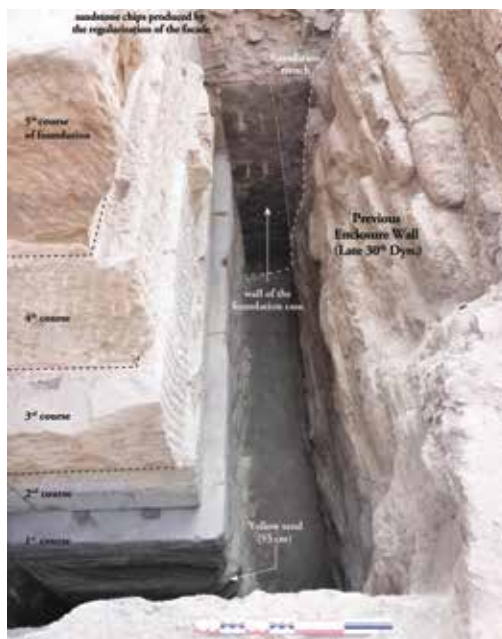
Figure 15. The deep trench on the northwestern corner of the Roman mammisi, showing the foundation techniques and the previous Late Period enclosure wall cut by the foundation trench (photo: G. Marouard)
