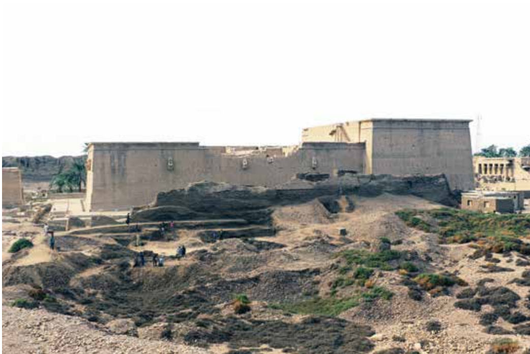
Figure 9. Ongoing cleaning operation on the eastern face of the early Middle Kingdom enclosure wall with the Hathor's temple in the background (photo: G. Marouard)
