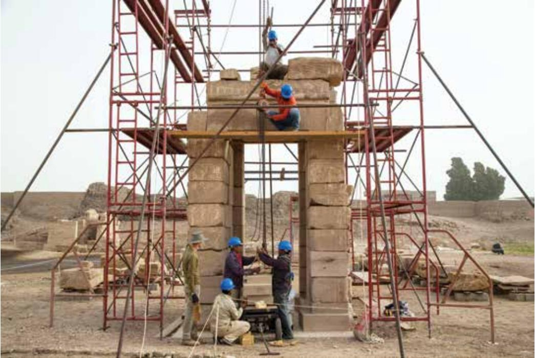
*Figure 16. Johannes Weninger and Chicago House workmen reconstructing the Domitian Gate, Medinet Habu (photo: Ray Johnson)*
