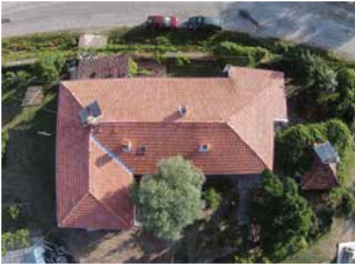
Figure 14. The new roof on the excavation house
