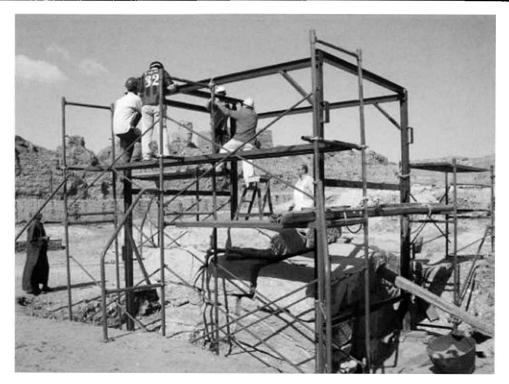
Erecting scaffolding over the southern well in preparation for dismantling
