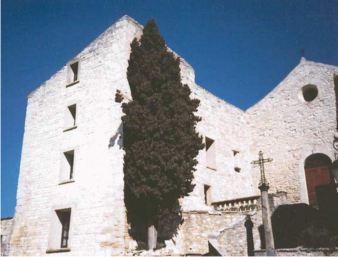
(c) The tower w/ staircase and door to church.
