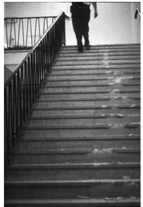
Figure 5. Staircase leading from the upper story of the Iraq Museum, its steps chipped by the weight of dragging a heavy statue from the gallery. Photo courtesy of McGuire Gibson
