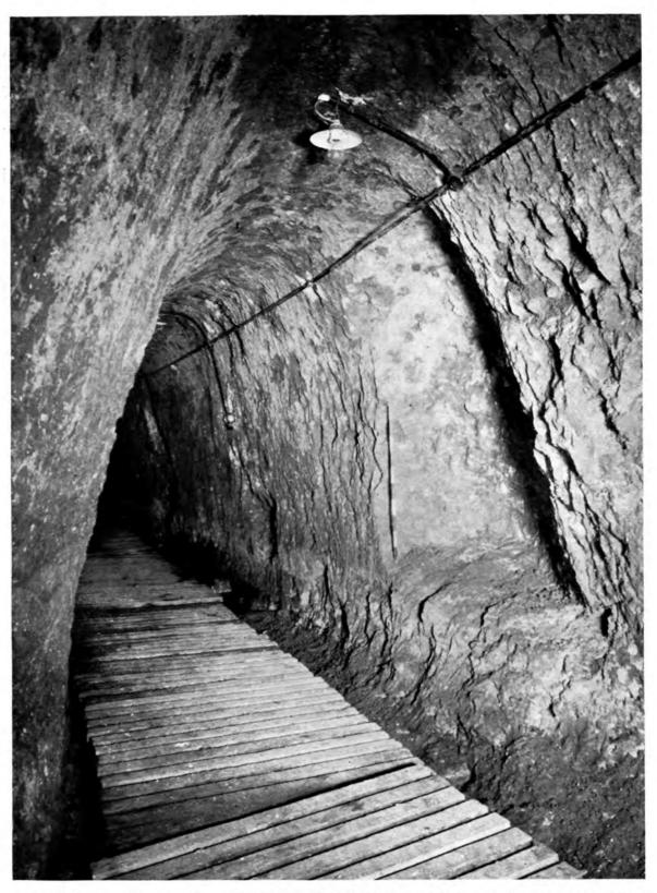
Fig. 15.—Indentation in the South Face of Tunnel 1000, Marking the End of the Western Section Where It Joined the Eastern Sounding Tunnel
