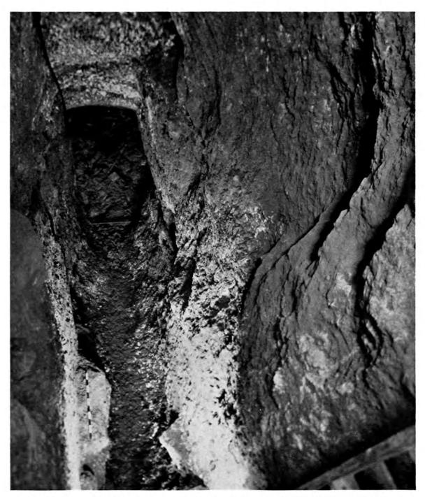
Fig. 20.—The Eastern Tunnel (1845) below the Masonry Stairs of the Inclined Passage (1116), from Above The meter stick rests on a remnant of the destroyed roof over the tunnel. Remains of four rock-cut steps of the original inclined tunnel are visible at right.
