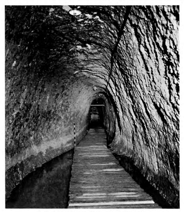
Fig. 26.—Tunnel 1000, Looking East toward the Inclined Passage The irregularity in the floor is a remnant of dam Y.
