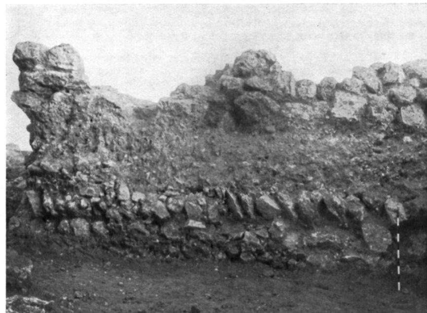
FIG. 77.—EXTERIOR OF SOUTH WALL OF TREASURY OBVIOUSLY NOT INTENDED TO BE EXPOSED ABOVE GRADE. FROM SOUTH
