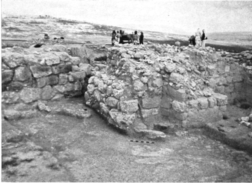
FIG. 65.—LOWER (VIII) AND UPPER (VII B) PAVEMENTS AT SOUTH END OF CITY GATE. NOTE VII B THICKENING OF SOUTHWEST BUTTRESS OVER LOWER PAVEMENT. EAST WALL OF PALACE AT LEFT. FROM SOUTHEAST
