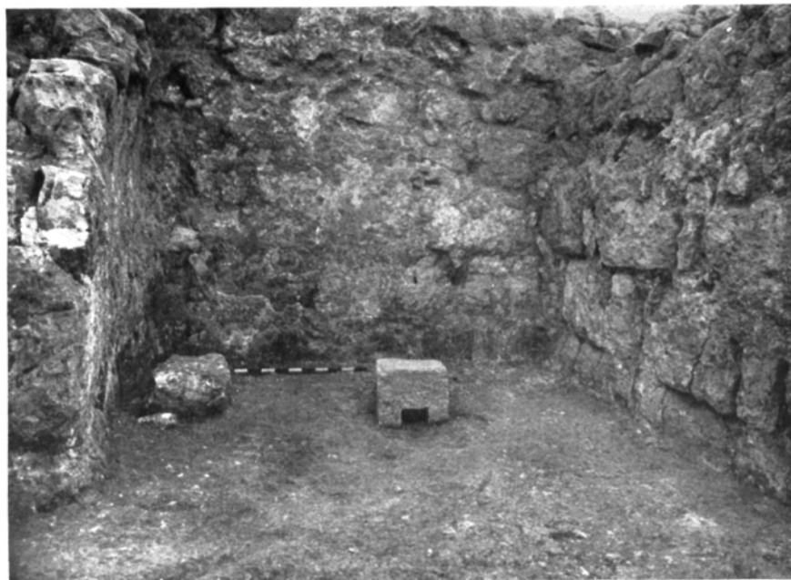
FIG. 78.—NORTH ROOM OF TREASURY SHOWING MASONRY WALLS PLASTERED TO A HEIGHT OF 3 METERS. FROM EAST
