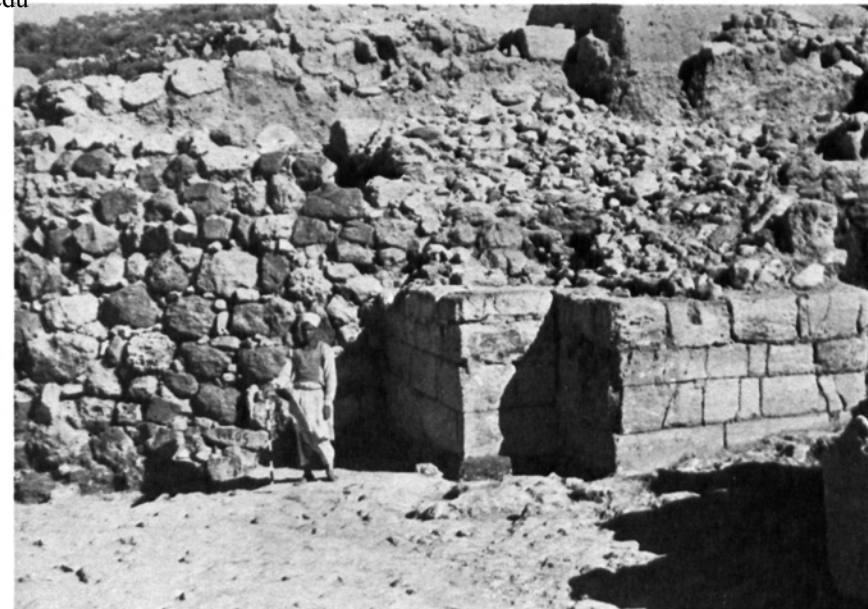
FIG. 44.—ASHLAR MASONRY OF OUTERMOST EAST PIER OF CITY GATE, NOTE INNER RETAINING WALL AT LEFT. STRATUM VIII. FROM NORTHWEST
