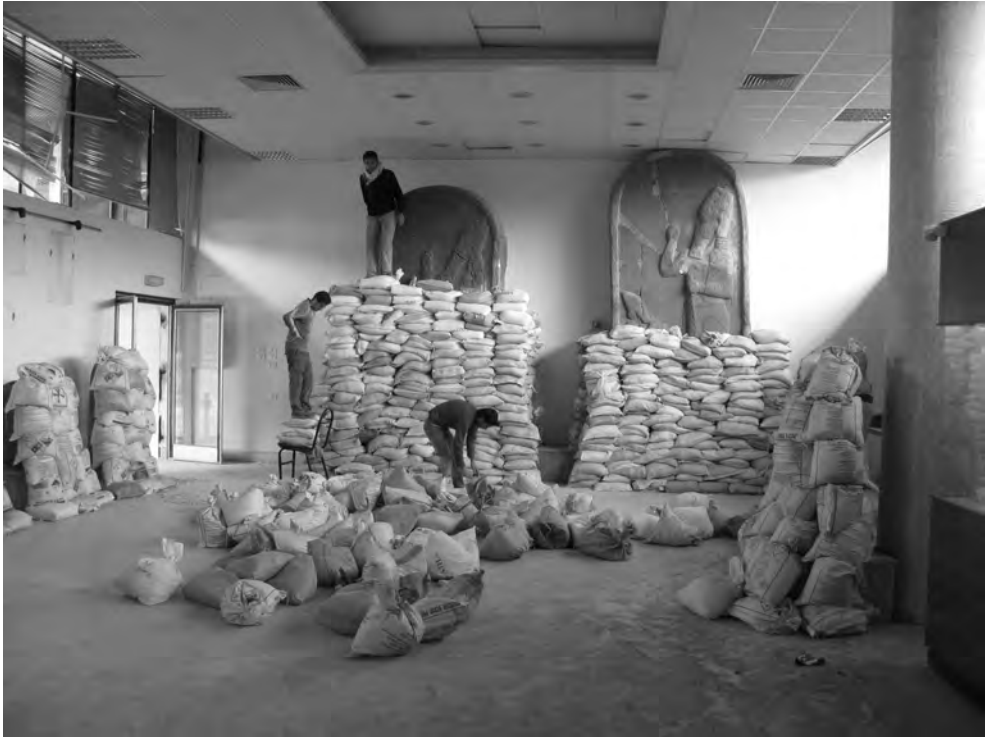
Fig. 3. The protection procedure of the large stela from Tell Ahmar at the Aleppo Museum.
