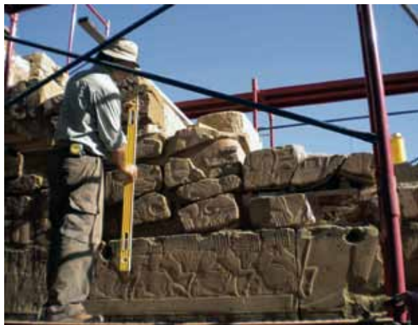
Amenhotep III outer wall slabs being mortared into place
