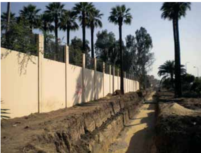
Service tunnel trench outside Chicago House, March 24, 2010
