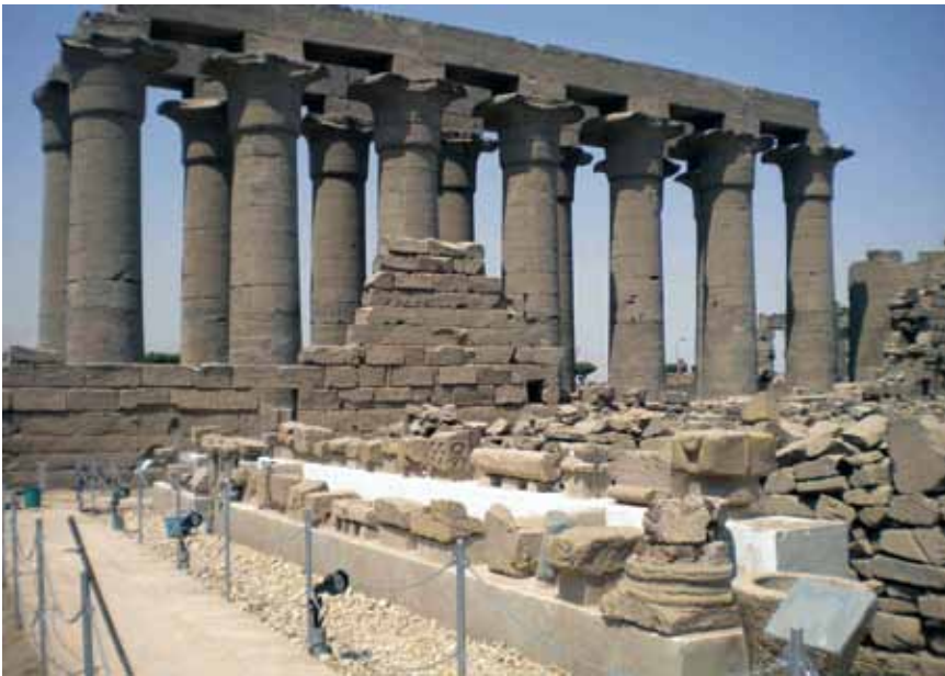
Dewatering display and Colonnade Hall
