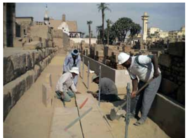
Luxor Temple blockyard open-air museum path construction
