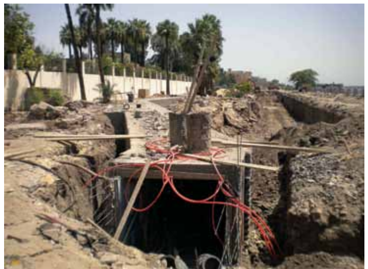
Corniche service tunnel and riverbank construction, June 2010
