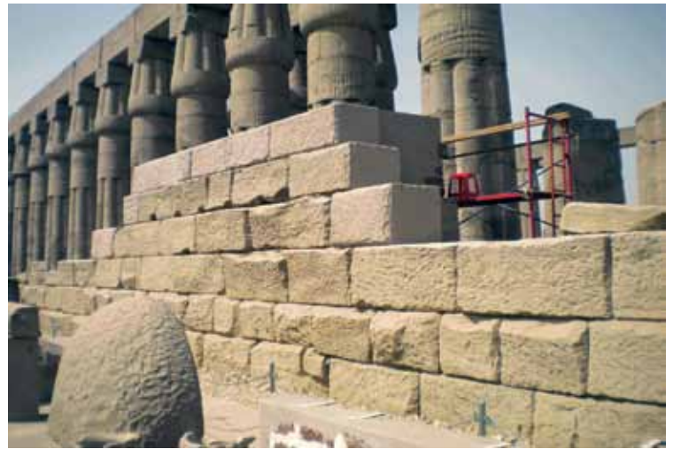
Amenhotep III outer wall finished
