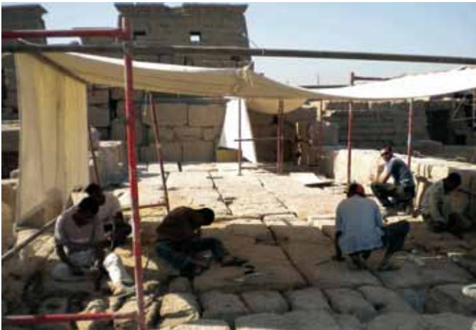
Khonsu Temple roof work
