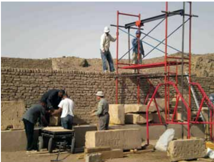
Medinet Habu blockyard block moving by Frank and crew
