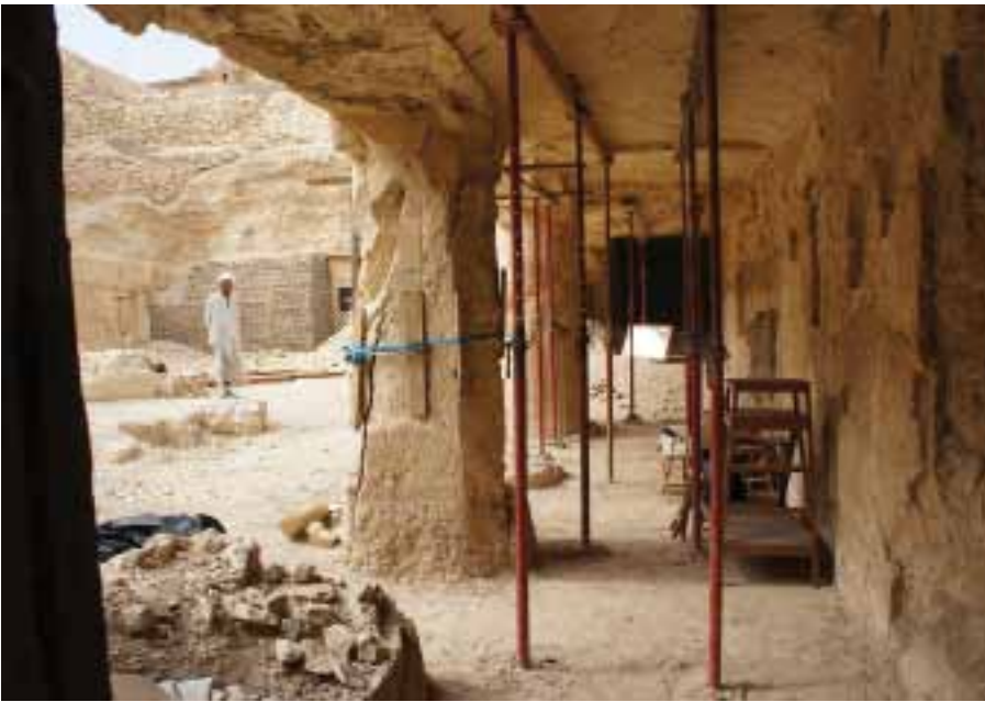
TT 107. Above: portico supported by screw jacks; top to bottom right: Sue drawing in TT 107; Margaret and SCA inspector Zenib at work, March 2011 (photo by Marie Bryan); and relief portrait of Neferssekheru
