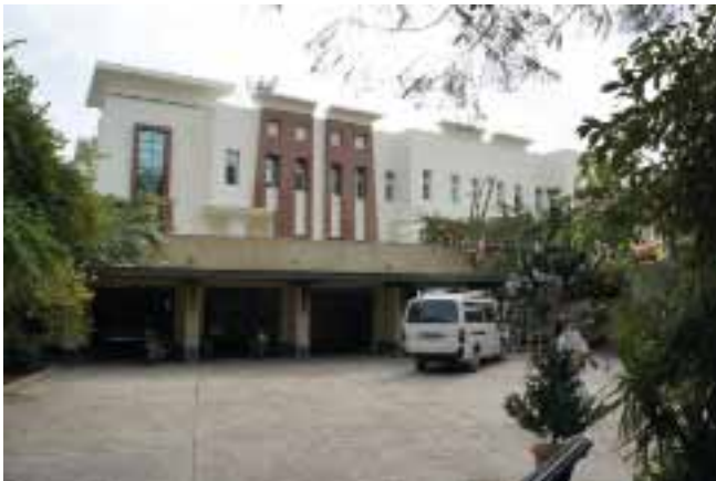
The new Telephone Central Office, from the front (top), and from the Chicago House back garden (bottom)
