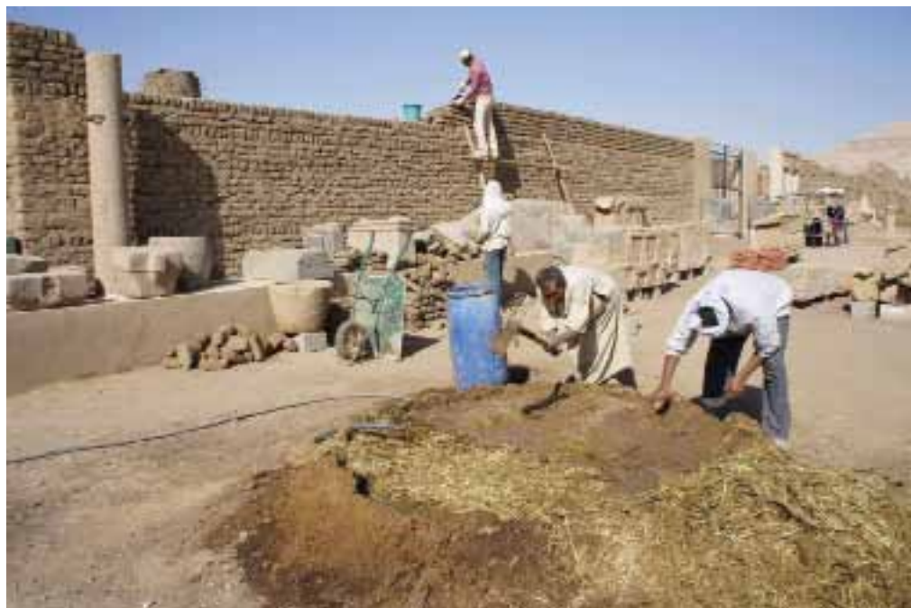
Medinet Habu new blockyard wall raising, March 2011
