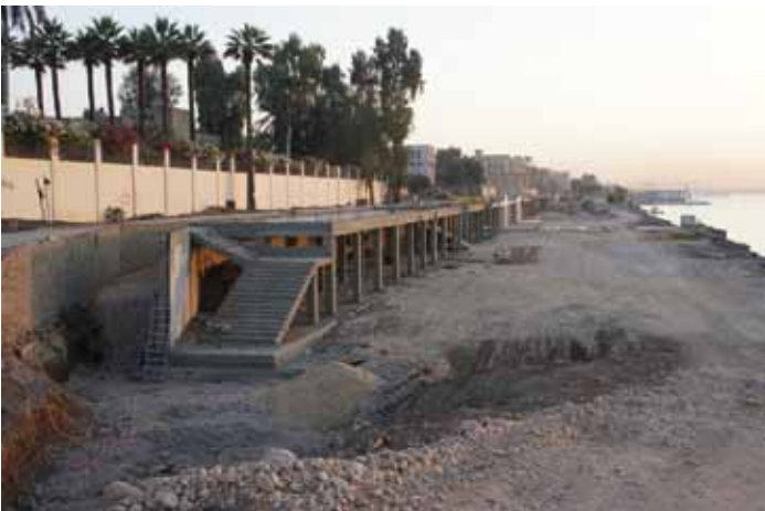
New pedestrian Corniche under construction, November 2010
