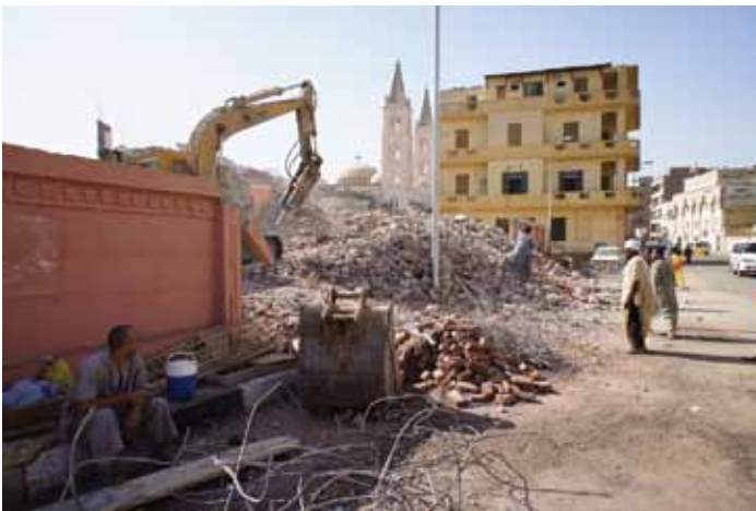
Apartment demolition, Karnak Street, late October 2010
