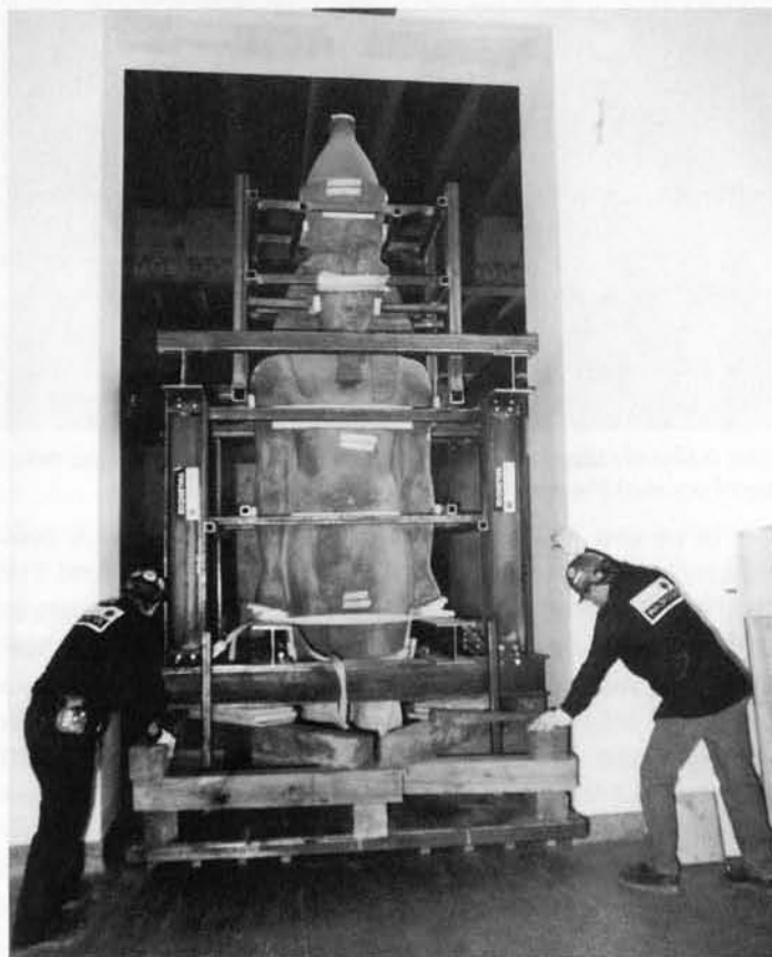
Left: Steel workers welding a steel cradle around the upper portion of the Tutankhamun statue to support it during its move to its new location
