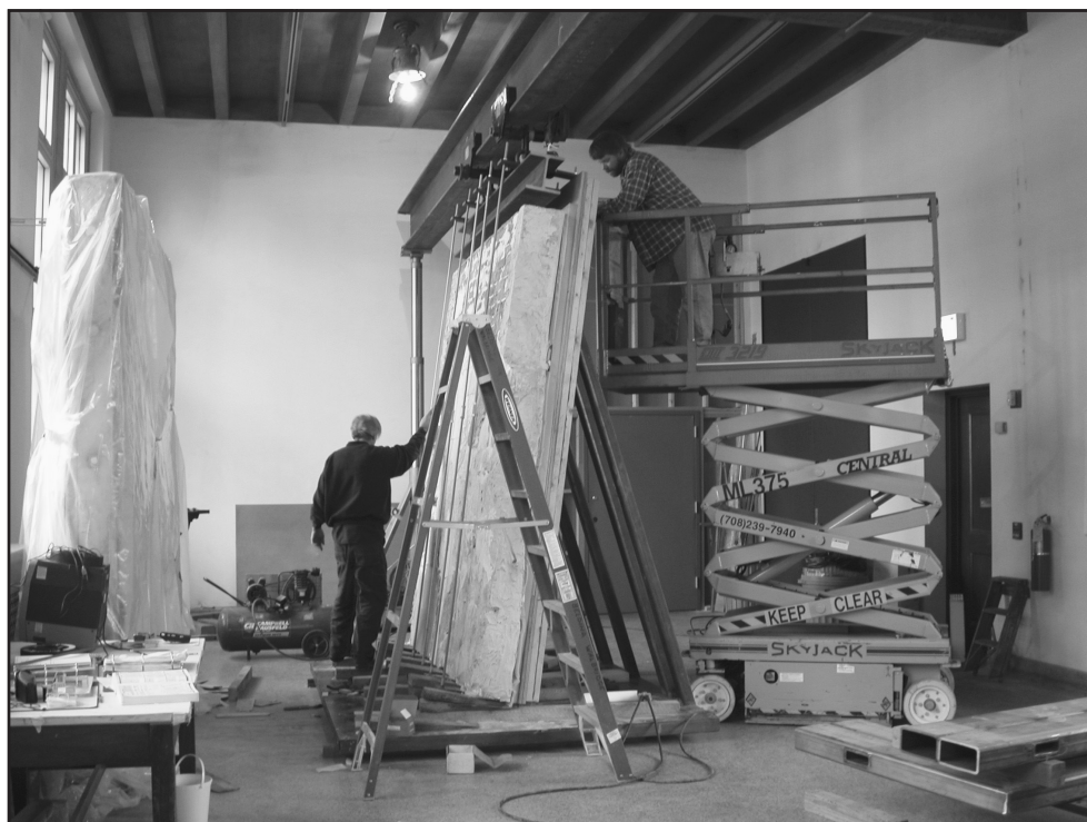
Museum re-installation continues as Belding Walbridge riggers begin the framing process of the next Assyrian relief in the East Wing. Photograph by Conservation Staff
