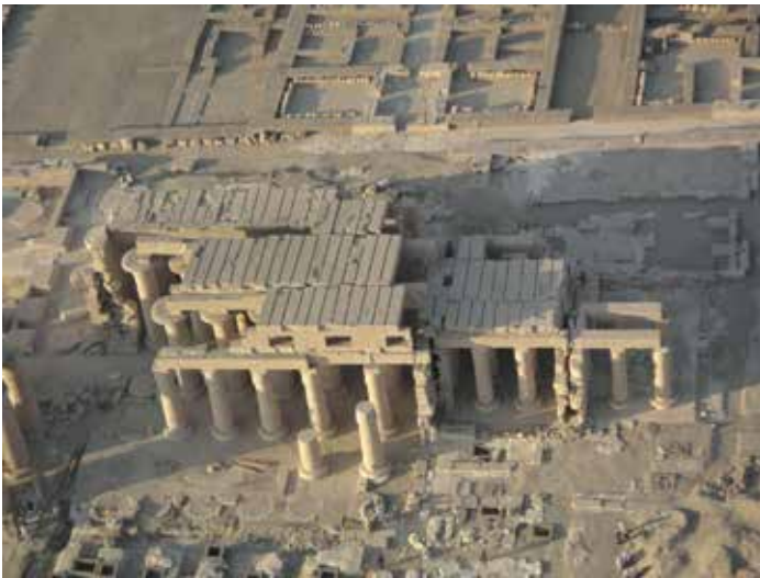
View of the roof of the Ramesseum from our hot-air balloon
